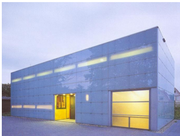
Figure 19: Dirk Jan Postel, Glass House in Almelo.
