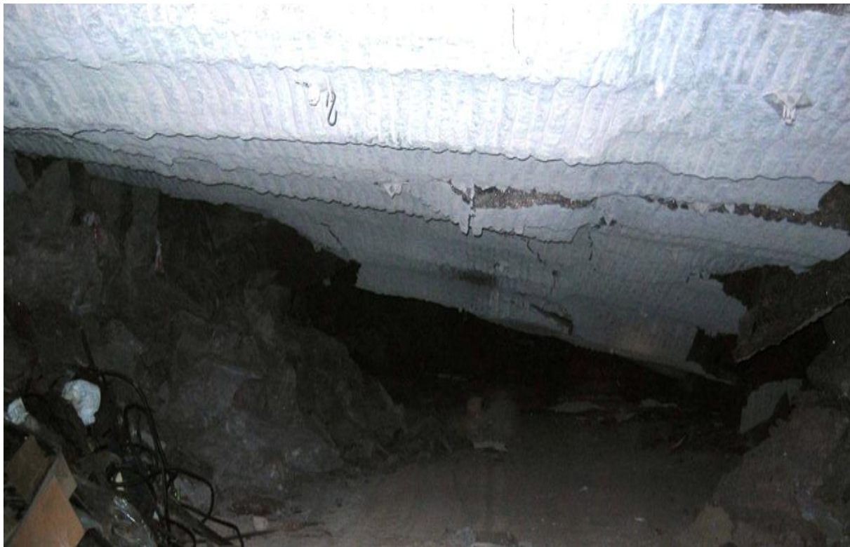
Plate 3.2 Closure in the underground working of Boulby mine in 2007. The roof has closed from over 3 m to less than 1.5 m in the foreground and almost completely in the background.
