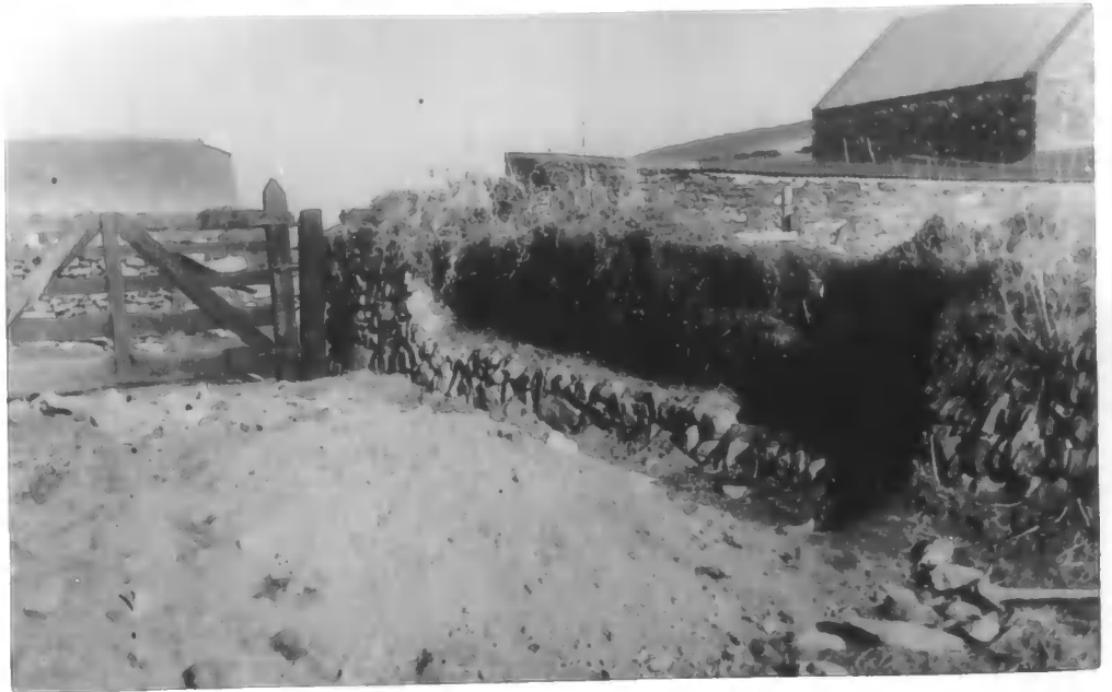
Plate 8. A Turf-and-stone wall in the course of repair in Cregneash, Isle of Man, March 1949. Photograph:- Manx Museum.
