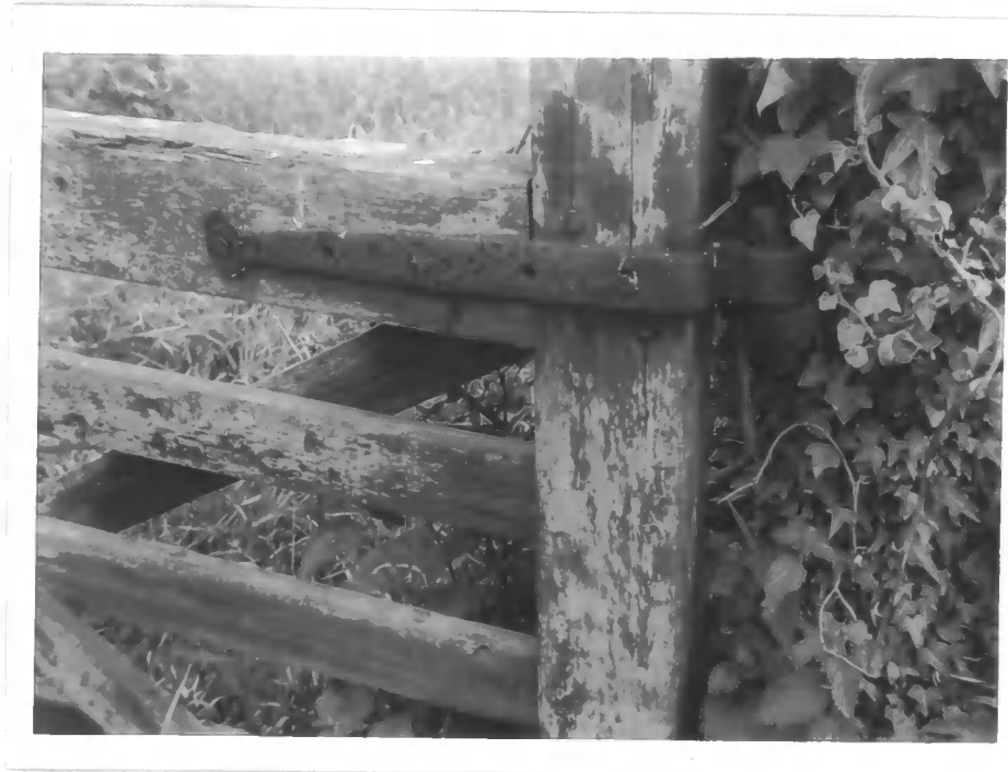
Plate 38. Ancient iron hinge on a gate near Downham Market, Norfolk. Photograph:- P. H. Armstrong.
