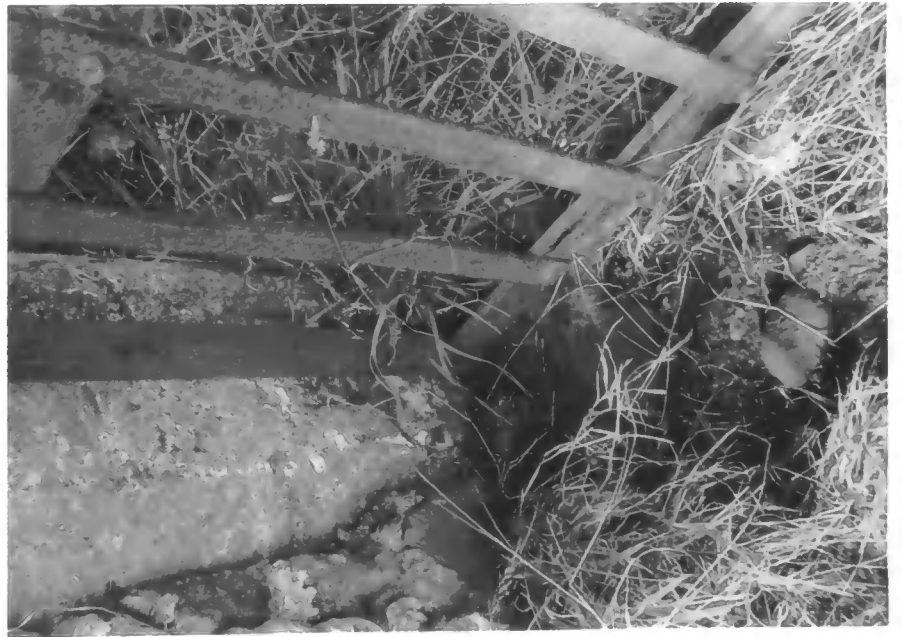
Plate 45. Harr of metal gate articulating in a spud-stone. Ballycastle, Co. Antrim, Northern Ireland, August 1964. Photograph:- P. H. Armstrong.
