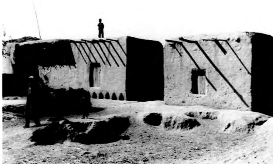
Grain stores raised above ground level to allow ventilation and avoid attacks by rats.
