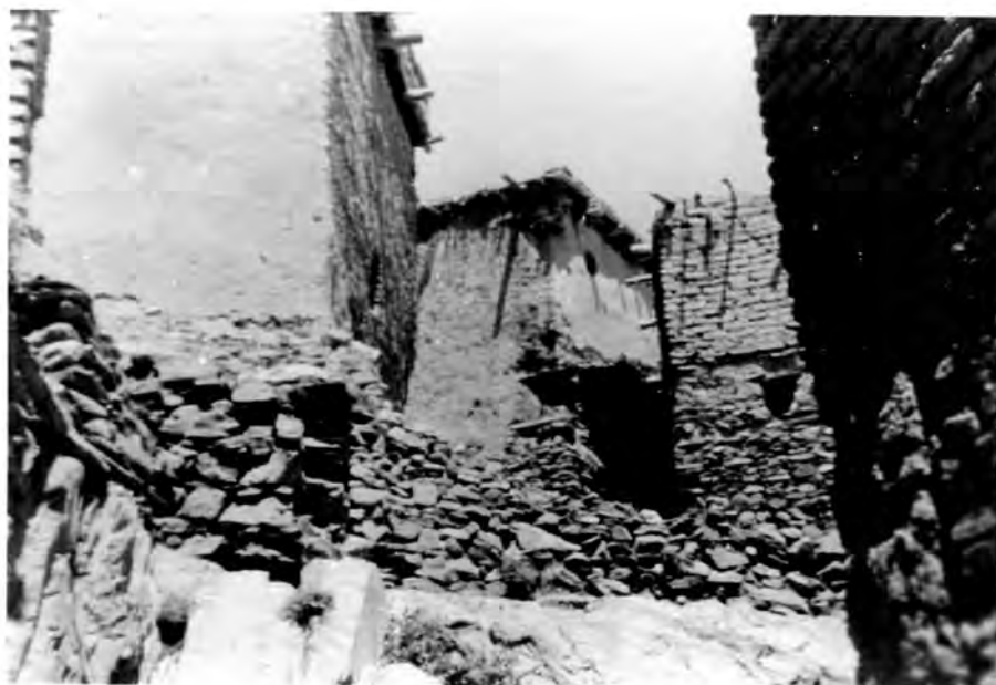
A predominance of stone interbedded with the clay is obvious in Khanrud.
