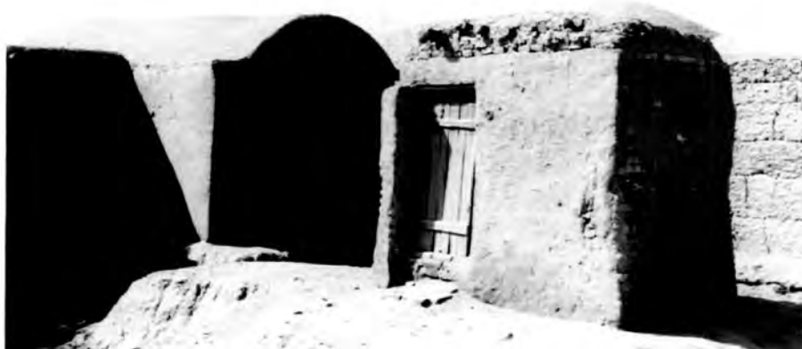
The two other principal types of roof found in villages on the plain are flat roofs and barrel roofs.
