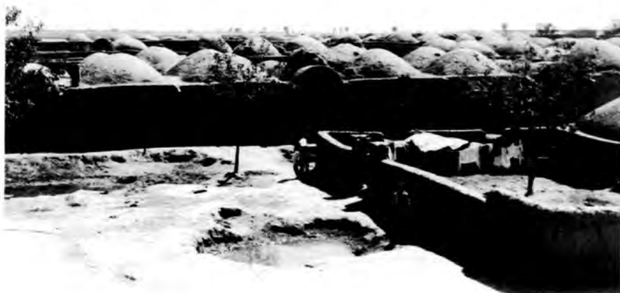
Semi-aerial view of a village typical of the plain; it is built almost entirely of sun-dried mud and its dome roofs are an extremely common sight.
