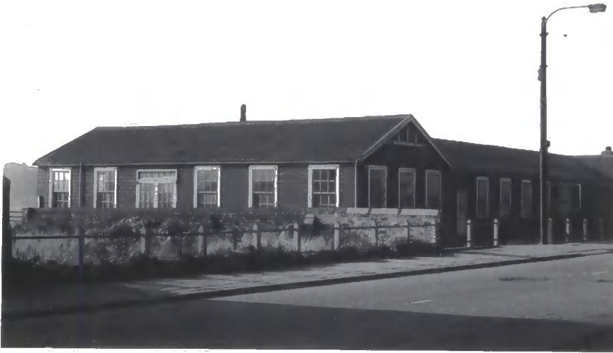
The Junior Instruction Centre at South Bank, opened 1935. The first to be built in England. Designed by the County Clerk of Works it cost £2,800 and proved to be most successful from a functional point of view. Timber built on brick pillars with asbestos roof.
