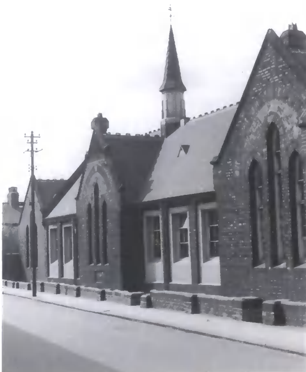
On left - South Bank Princess Street Elementary School. Built 1878. Thought to be a typical example of an unfortunate period of school architecture. Originally an all age establishment with three departments.
