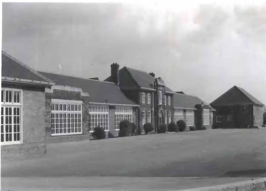
Sir William Worsley Senior Elementary School. Built 1936 The building incorporated 'Hadow' ideas.
