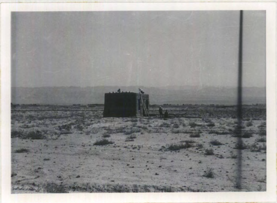
Haji Nasir - poles being laid on house walls before roofing with mud.
