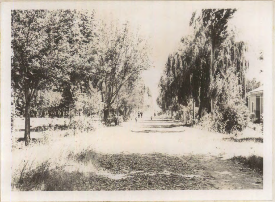
Haji Nasir - view along the main avenue towards the main entrance - the landlord's garden.
