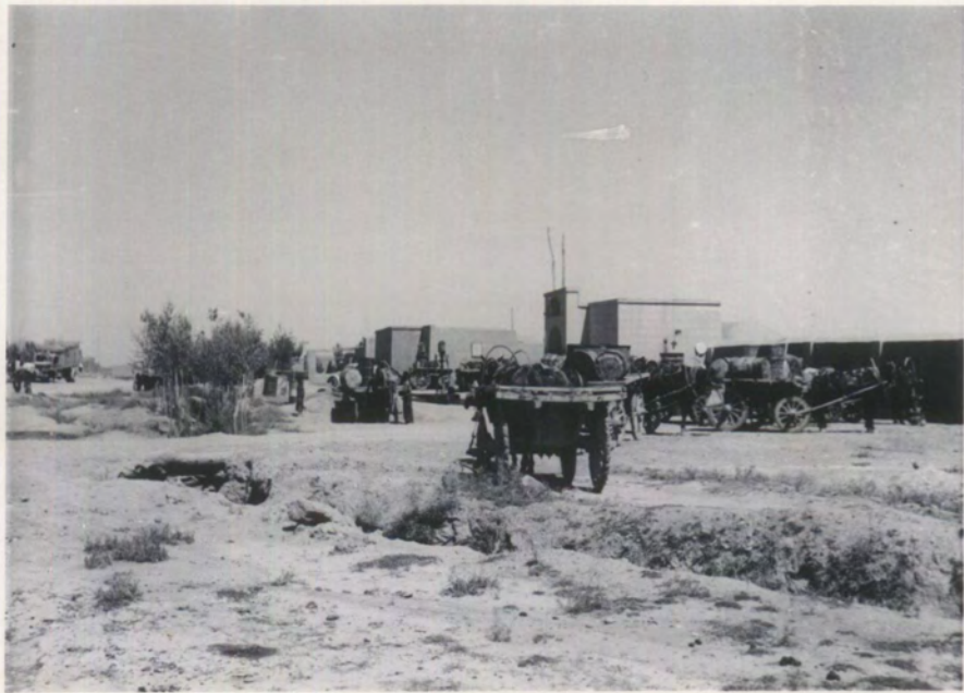
Haji Nasir - traditional carts opposite the petrol pumps in the new main road settlement.
