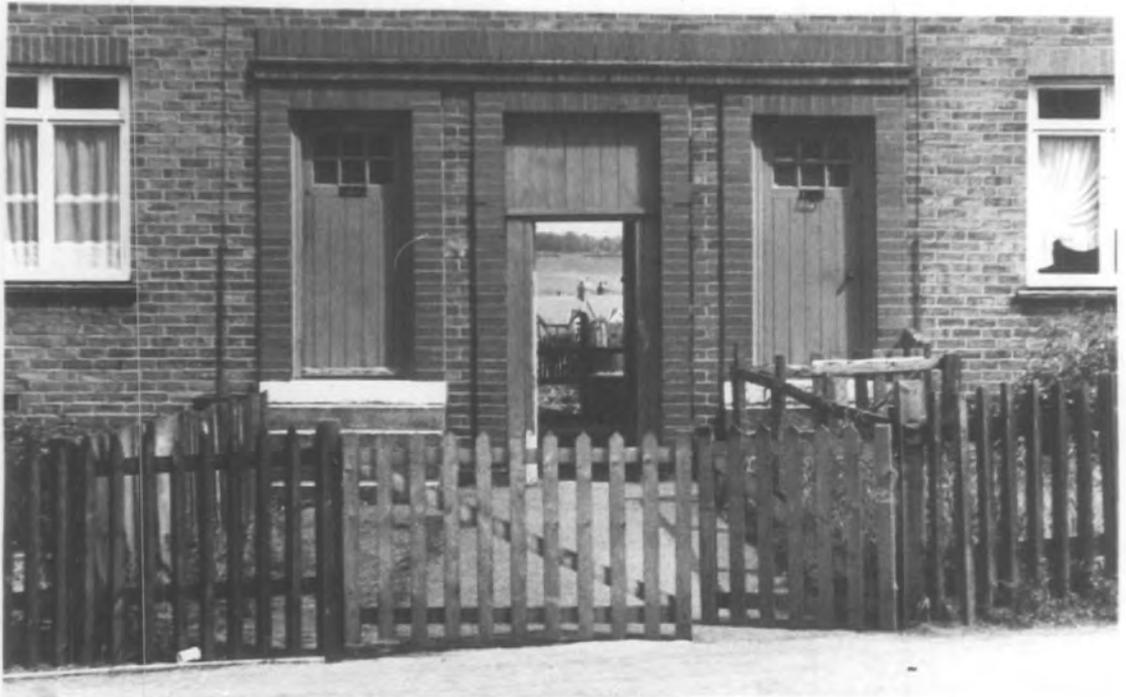
ILLUSTRATION 4-3 Pringle Place, New Brancepeth. A through-passage was the standard Tudor Walters method of improving rear access to blocks of four or more houses.
