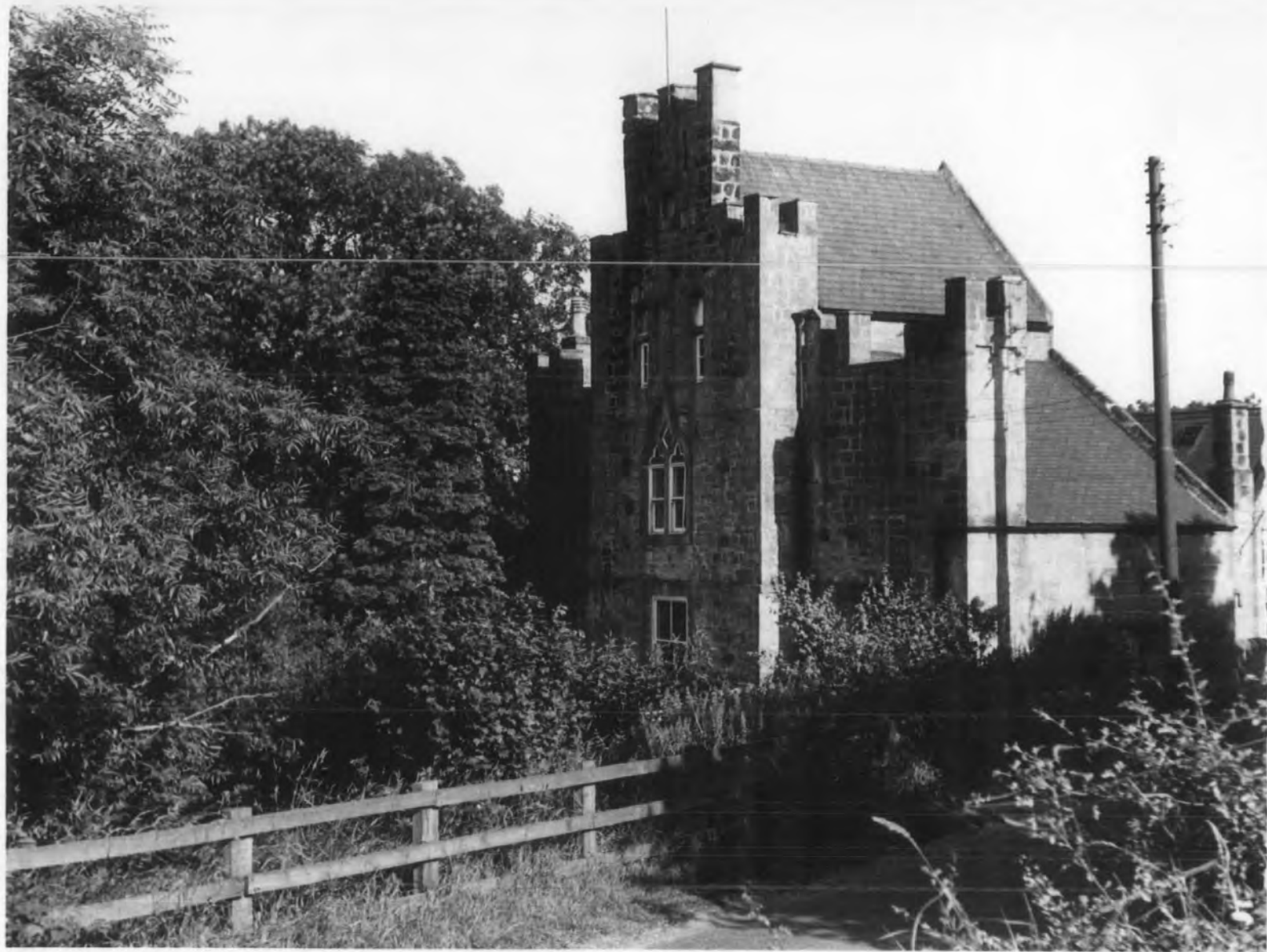
Plate Two. Hartburn village school, Northumberland built c.1750. Stables formed the lower storey with the school above.
