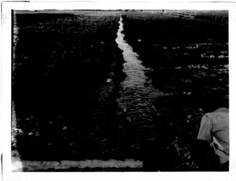
Plate 18(b) - Suqia - irrigation trench to distribute water for irrigation to the jedawel.
