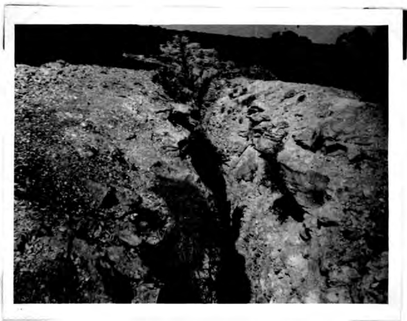
Plate 7(b) - The unfinished pipeline between Ain Mara and El-Marj.
