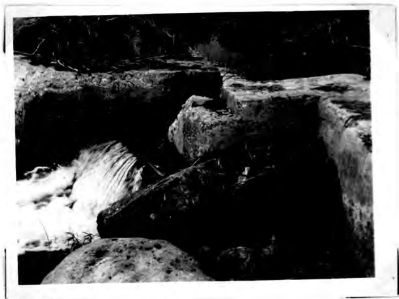
Plate 5(a) - Damage caused by the flooding of Wadi Derna to Ain Derna. December 1958.
