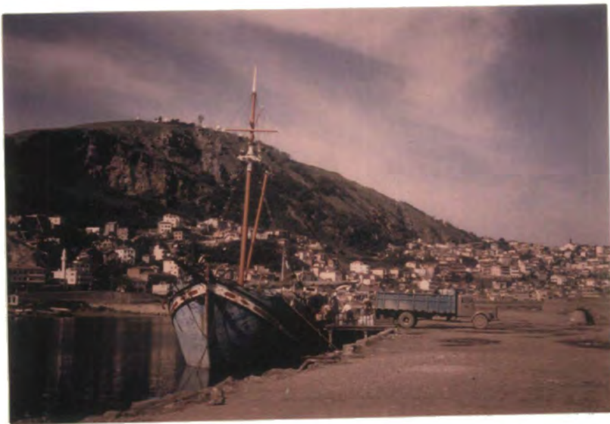
6 Trabzon, The old harbour. The andesite mass of Boztepe rises along a fault line behind the city.
