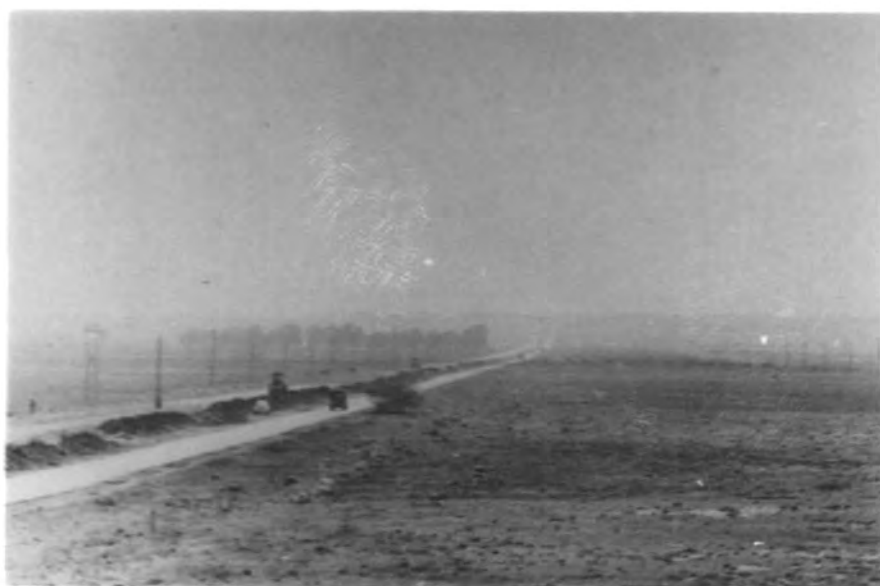
Plate 11.7. The new Benina dual-carriageway (under construction, 1967)
