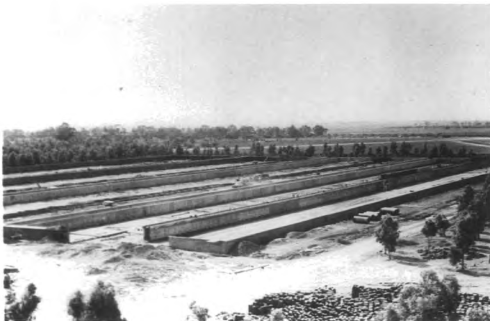
Plate 5.6. El Gwarsha Sewage Purification Plant (under construction, 1967)
