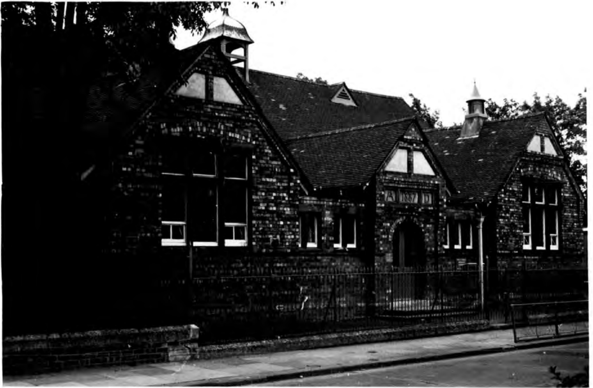
THE TWO SCHOOLS BUILT IN WEST STREET BY THE L.N.W.R. COMPANY
