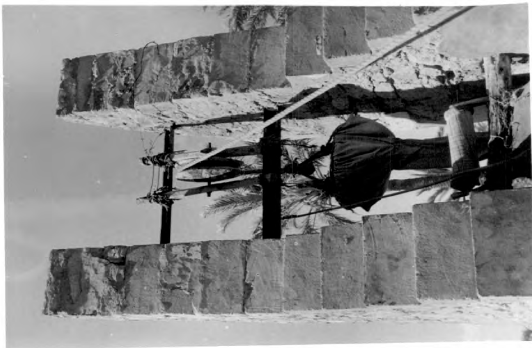
ABOVE Well superstructure, pulley system and dalu water lift. Location - Sahel El-Ahamed.
