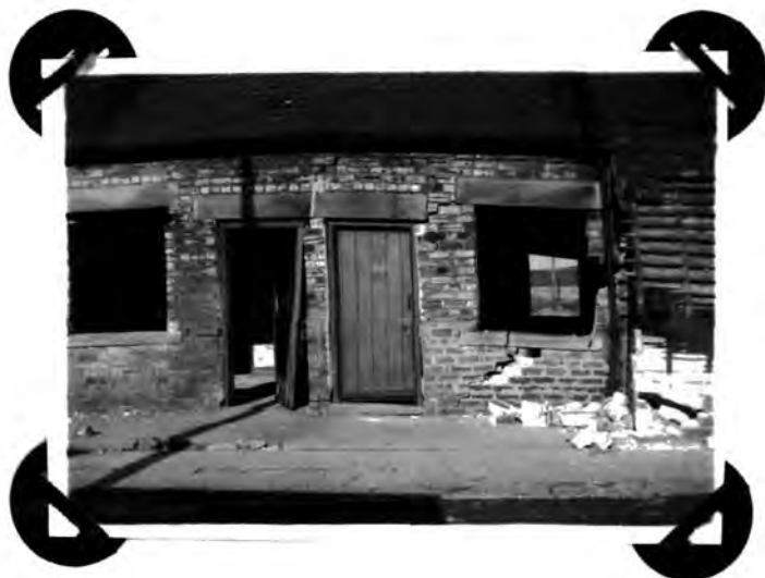
Damage caused by subsidence.
