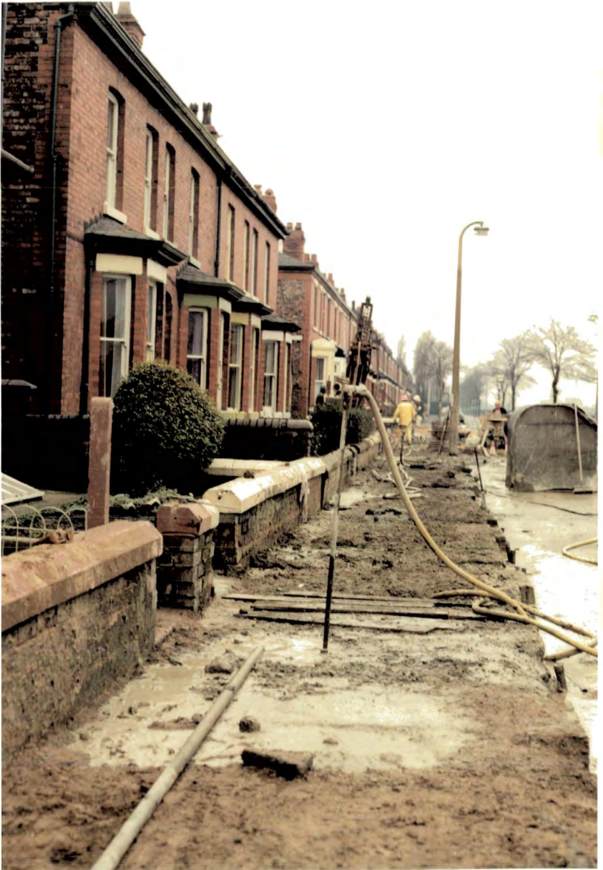
Plate 6.4 Nos 29-32 ELLESMERE Rd DURING GROUND TREATMENT
