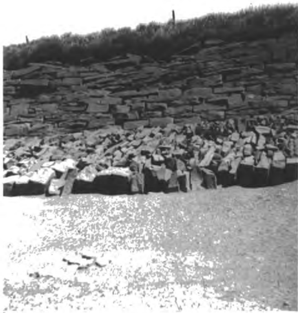
Photograph.11. Station E on 12.6.57. Note sandy bottom and horizontal flange at base of wall.
