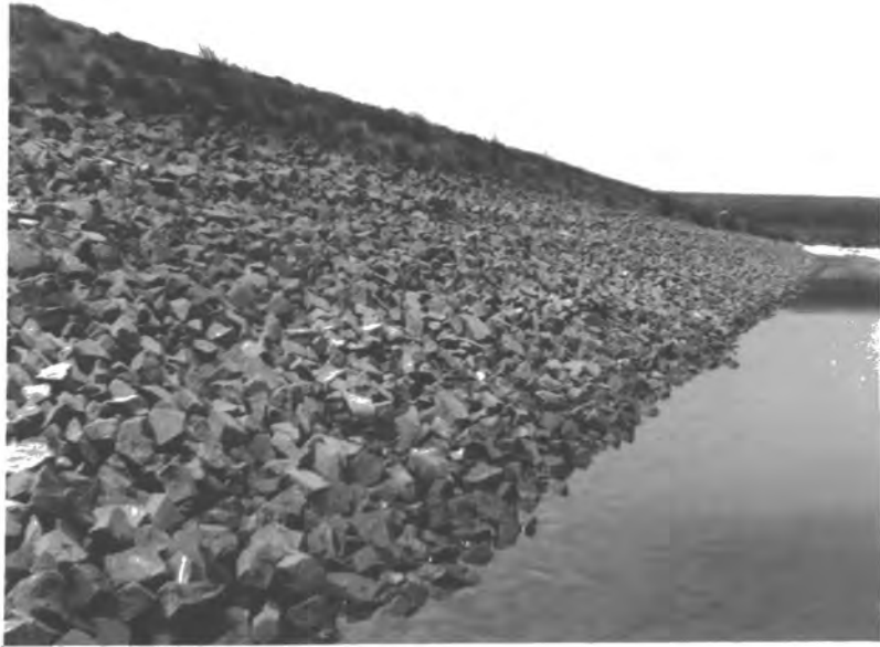
Photograph.7. Stony bank on section A100 to A300,12.6.57.
