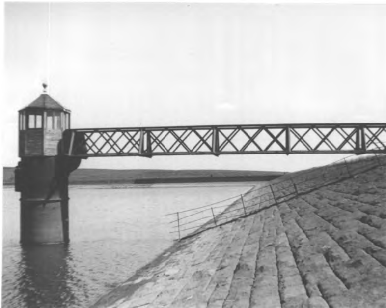
Photograph.5. Tower on 12.6.57. Top water level is just below the flange on the base of the tower. Distance from flange to water level shown is about 5 ft. (1.5 m.).
