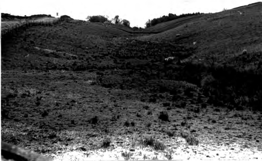
Channel k (Fig. 5.5) - view looking south.
