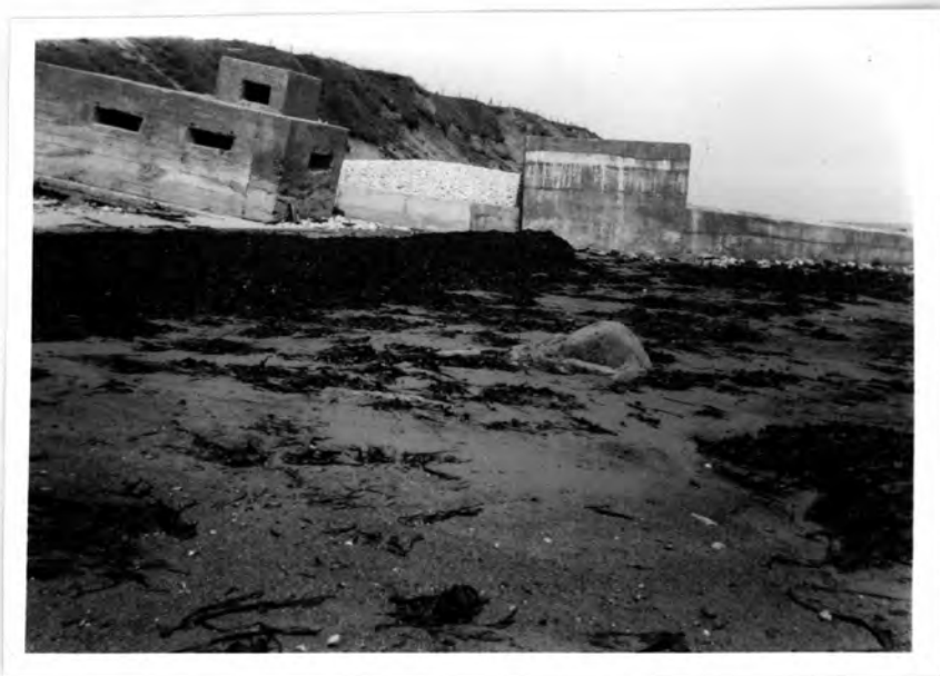
Plate XIX: The construction of a new sewer outfall at Whitburn has resulted in much shingle and sand accumulating immediately to the north and a comparative shortage of such material to the south. In places the height difference between north and south beaches is about five feet.
