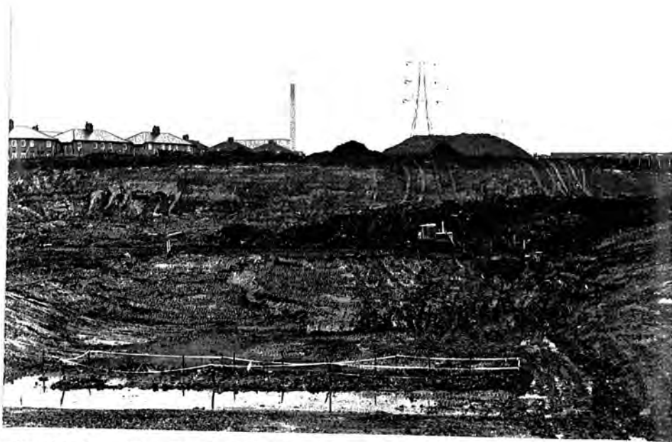
Plate 10.2 The Floor of the Partially Completed Excavation at Howdon Viewed Northwards
