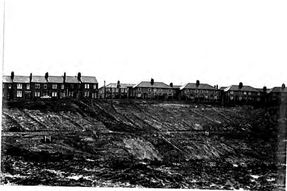
Plate 10.1 The Western End of the Excavation Underway at Howdon
