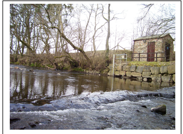
Figure 2.3 Dacre Bridge gauging station.
