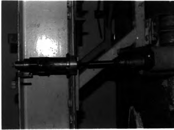
Applying pressure using ordinary 2 ton car jack
