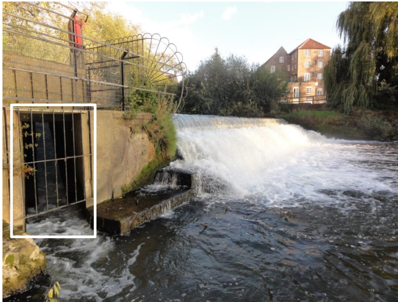
Figure 2.3. Stamford Bridge weir. The white outline indicates the location of the Denil fishway entrance. Photograph taken on 07/10/2011.
