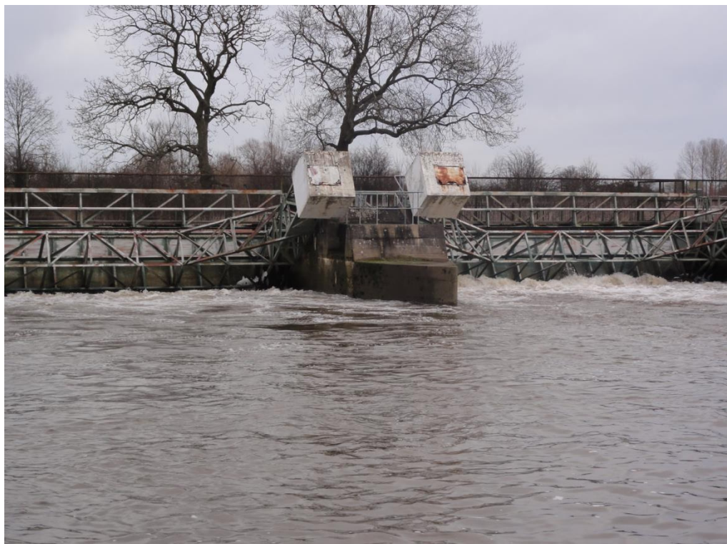
Figure 2.10. Elvington Sluices in flood conditions on 14/02/12 (mean daily flow 30.7 \text{ m}^3 \text{ s}^{-1} ).
