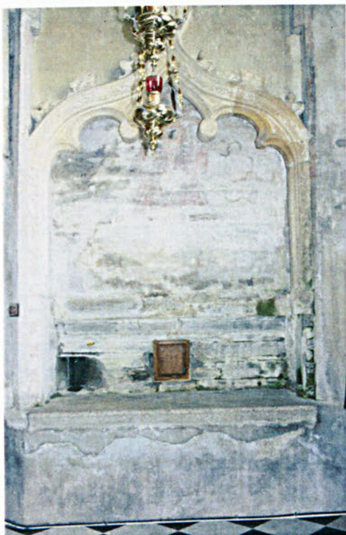
Fig 5.6 Shrine structure illustrating surrounding frame, ogee arch, stone casket, recess with wall painting, wooden aumbry and squint.
