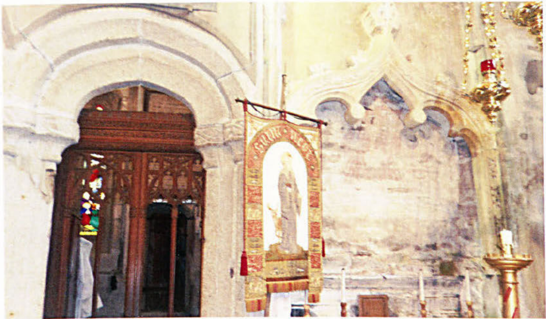
Fig 5.4 Arrangement of shrine and north chapel doorway northern resulting in the truncation of the northern arcade bays
