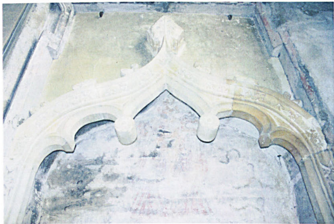
Fig 5.8 Ogee arch detailing carving, different geologies of stone and polychromy on jamb.
