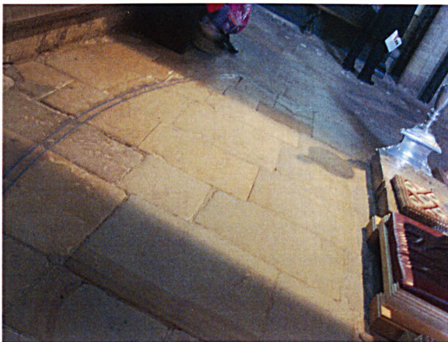
Fig 4.2 Termination line of original apse shown on current feretory pavement, Durham Cathedral
