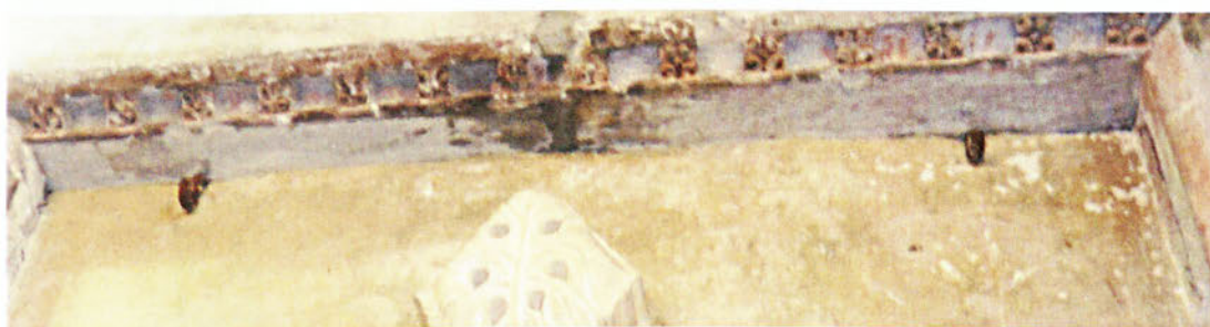
Fig 5.23 Iron hooks located at top of frame surrounding St Neot shrine
