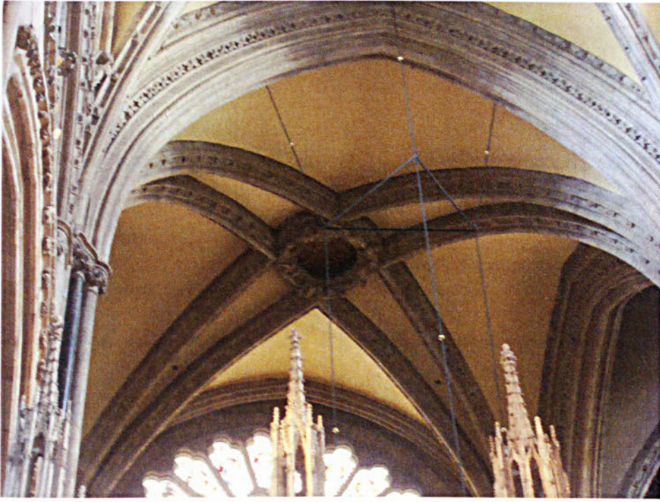
Fig 4.5 Star pattern made by cross-ribs of feretory vault.
