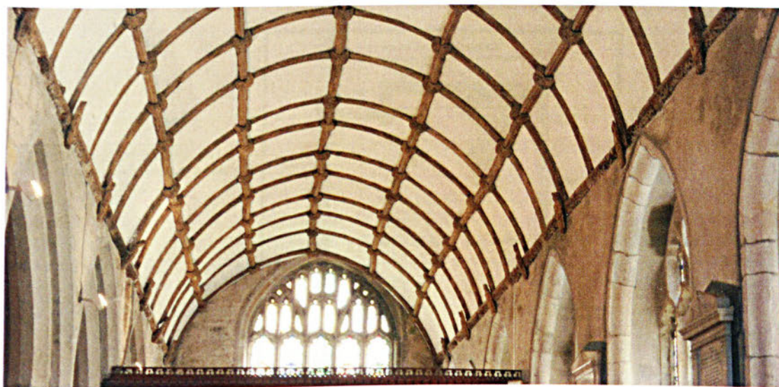
Fig 5.31 Wagon roof, St Neot
