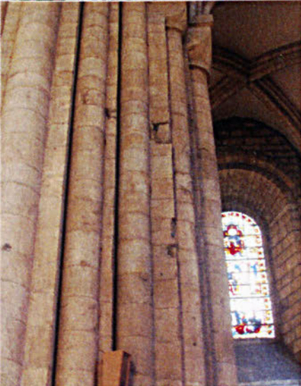
Fig 4.32 Grooves and rectangular holes in piers, nave, Durham Cathedral.
