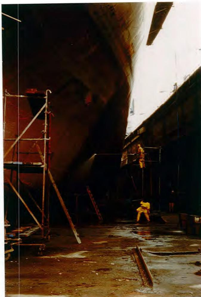
Figure 1.24 High pressure water cleaning of a vessel in dry dock
