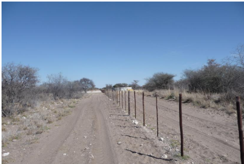
Figure 2.6 Typical five-strand cattle fence
