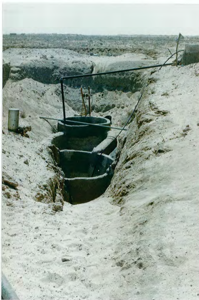
FIGURE 3.3 : Reconstruction of an old well
