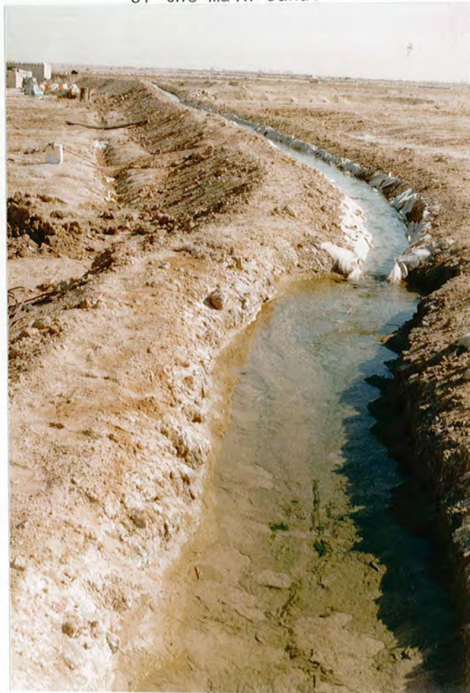
FIGURE 3.7 : Use of plastic sheets to line some portions of the main canal
