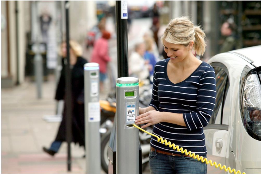
Fig 1.4 An Elektrobay recharging pillar. (By kind permission of Elektromotive Ltd)
