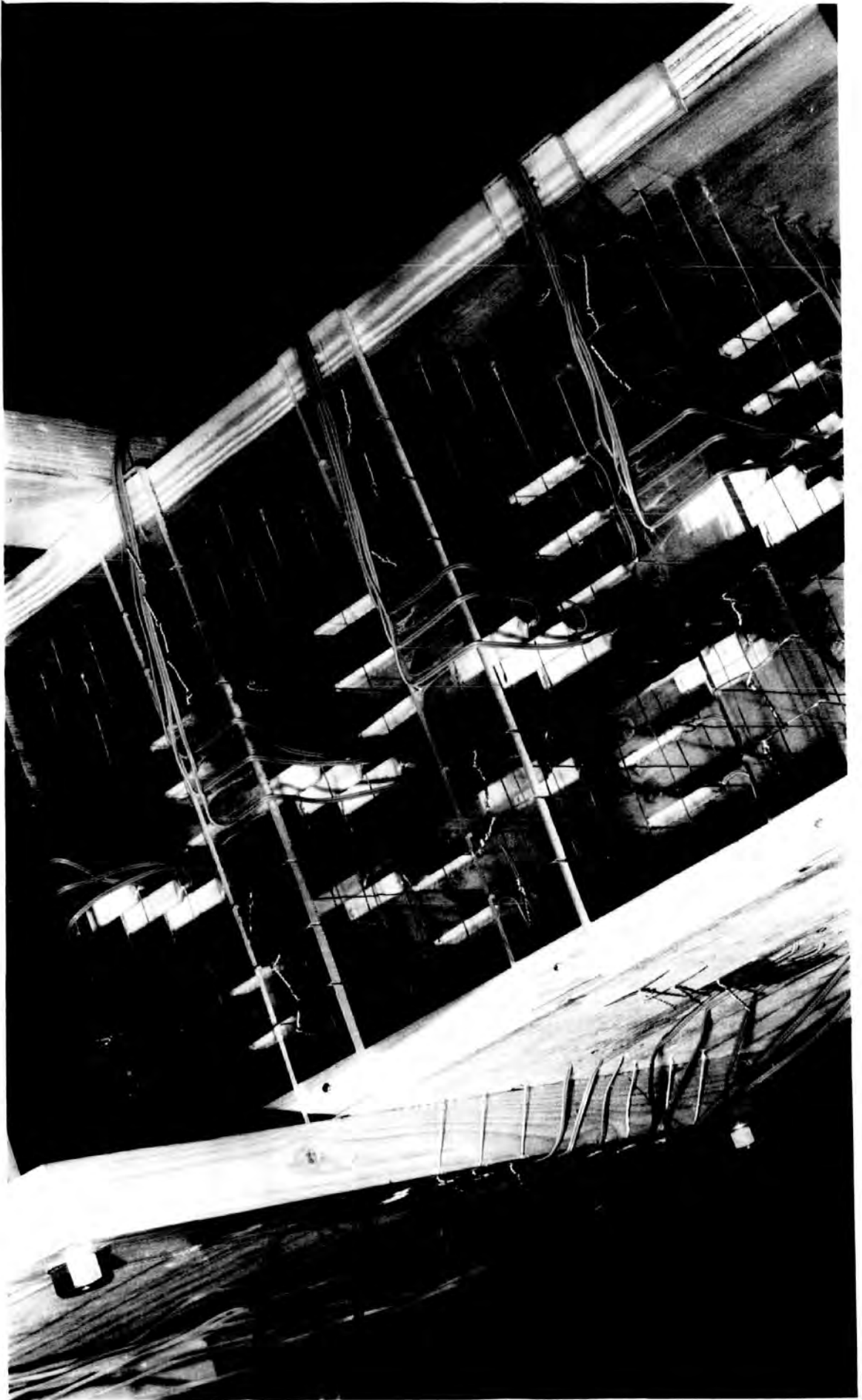
Figure 9.6: Embedment Gauges (Specimen 200T20)
