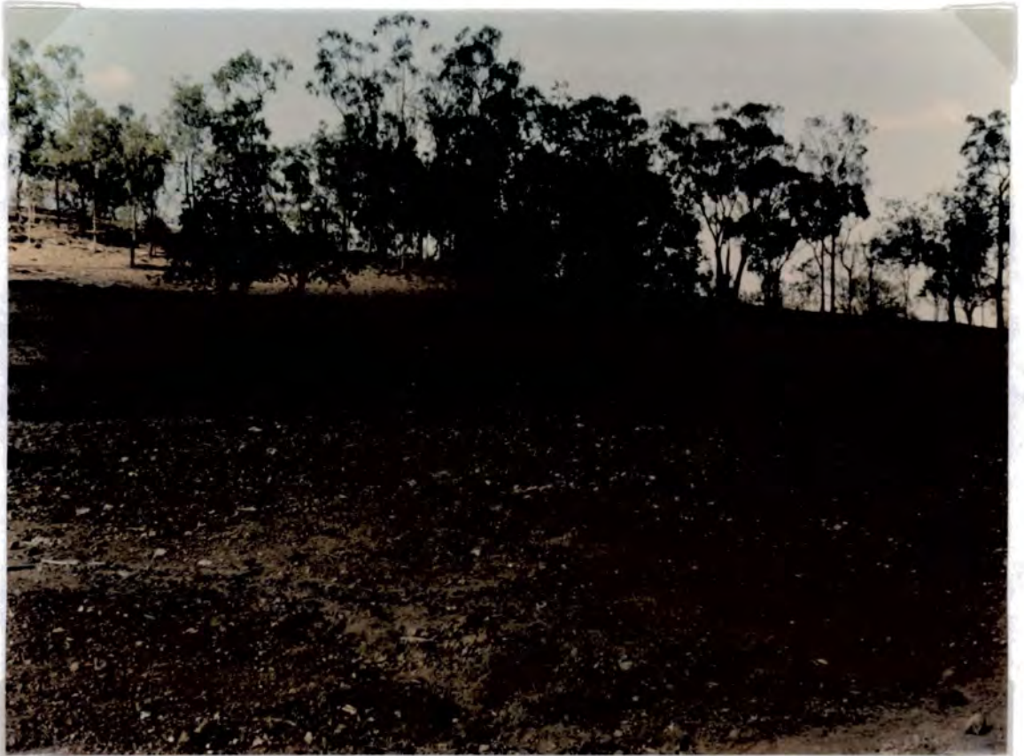
Plate 5.4 Location 2 at Pinnacle creek (Site 1). This area is underlain by the volcanic breccias. They are heavily weathered, little outcrop is evident. Note the very thin vegetation cover and the extensive scattered rock debris.
