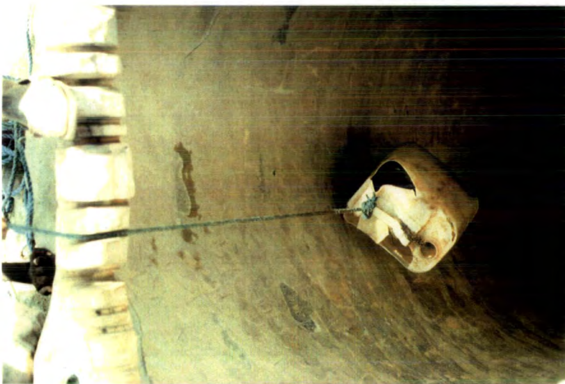
Plate 32: Water is raised by a man using an 'open-topped' jerrican attached to a rope at Wakeel. The rope is pulled over a highly-grooved branch.
