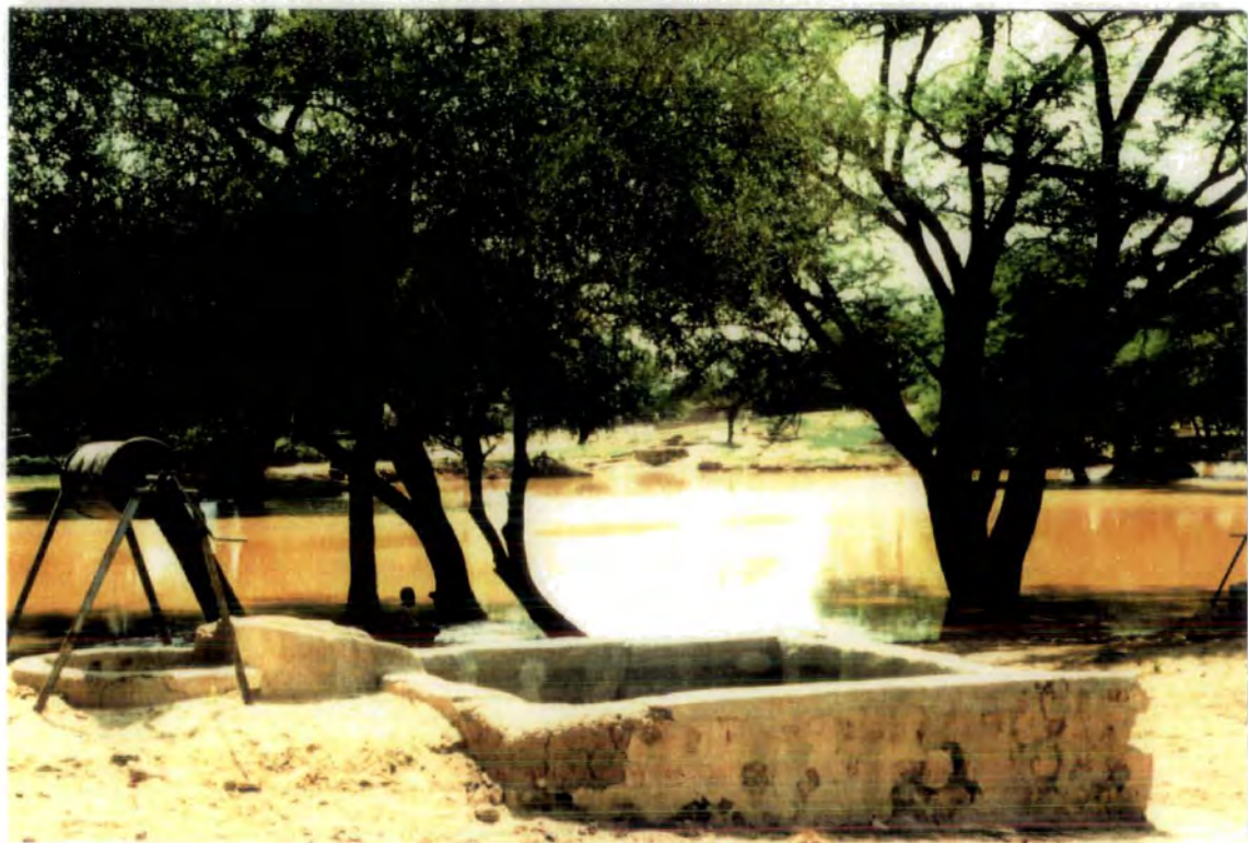
Plate 15: A well at En Nahud town located next to a tree-lined fula. A windlass system is installed and there are cement basins and chutes to aid distribution.
