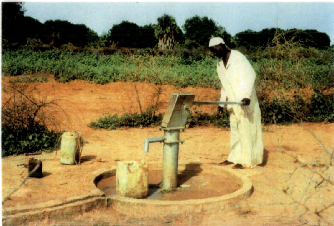
Plate 19: A UNICEF handpump near Er Rahad is simple to use. Wastewater is collected and channelled outside a small enclosure.
