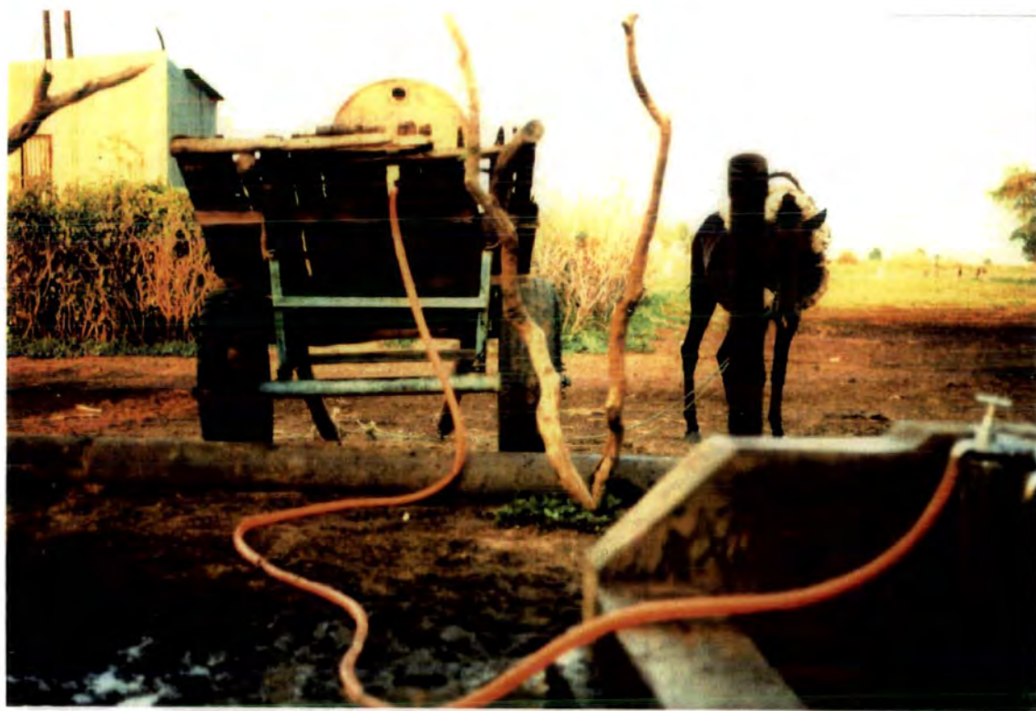
Plate 9: Caros commonly filled within the wateryard area by fixing a hose to taps at tapstands, as seen at Khammas Hajar.
