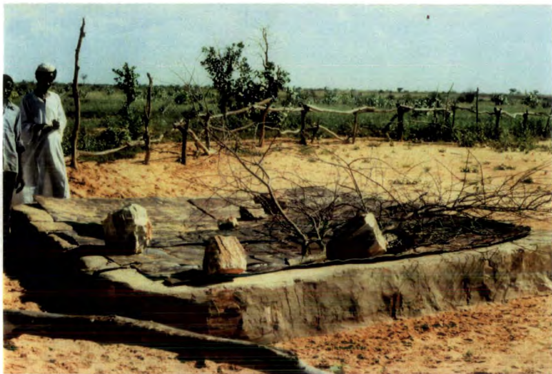
Plate 25: The cistern at Abu Shura with a metal cover weighted with stones and in a fenced enclosure.
