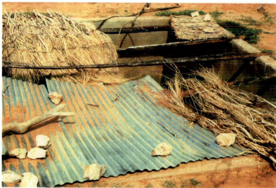
Plate 26: Part of the metal covering at the cistern at Umm Bum was sold and a thatch one constructed in its place. As a consequence the water was considered unfit for human consumption.
