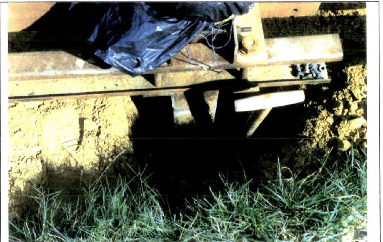
Plate 3.6 Excavation of sand around a pile.
