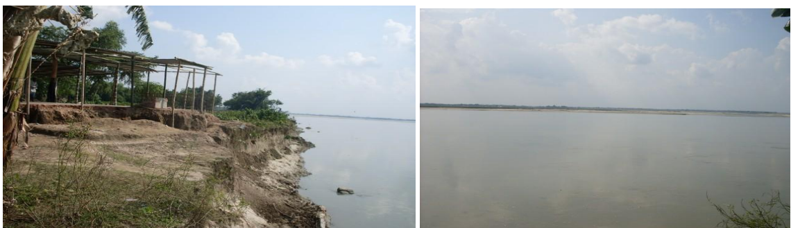
Fig 4.2a: River bank erosion and a collapsed mosque in Kismat Batrigach enclave (top); some of the residents of this enclave could still identify their previous houses were somewhere in the middle of the present river (bottom).
