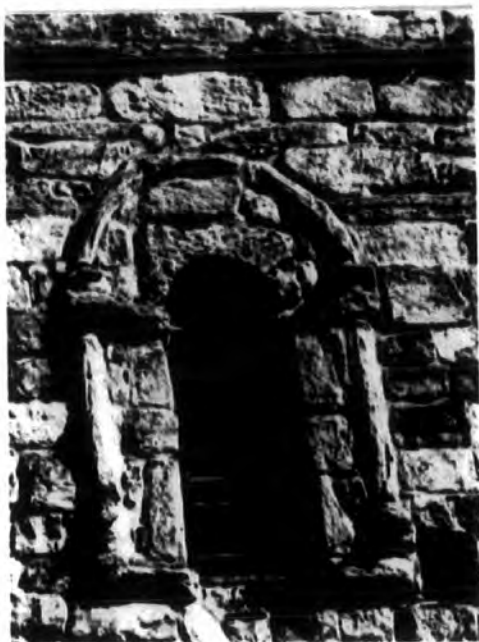
Detail: upper doorway on south
