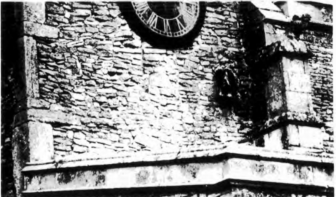
Detail of tower's south face: blocked opening
