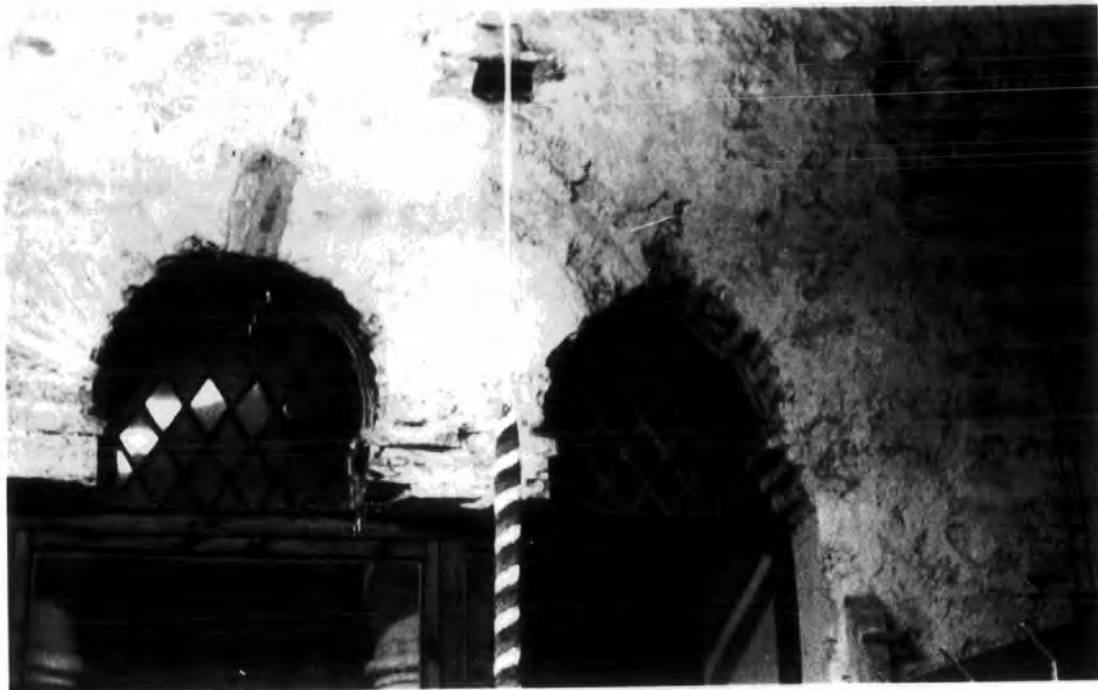
First floor chamber interior: windows to nave, detail
