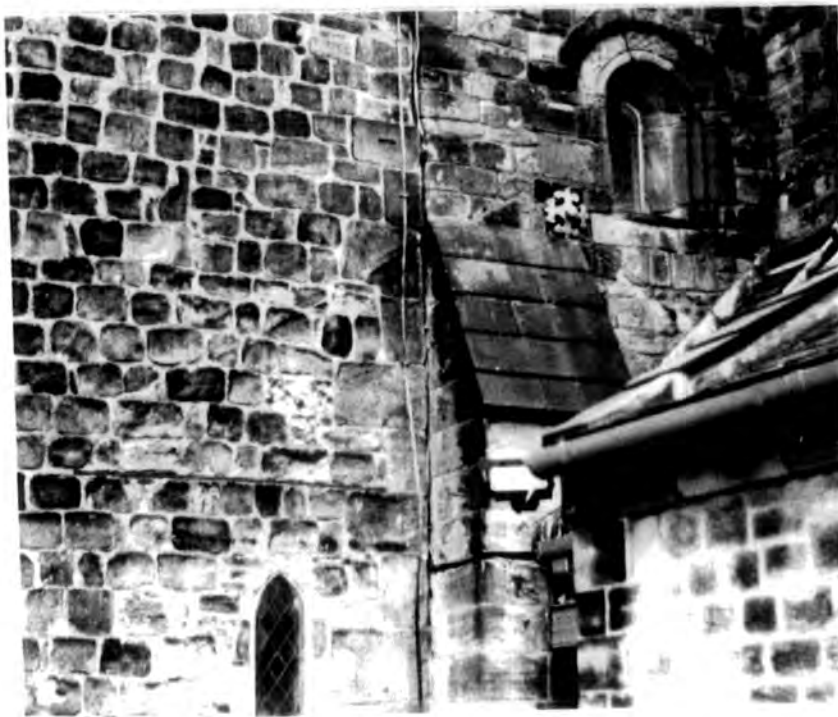
North wall: tower window and gable lines
