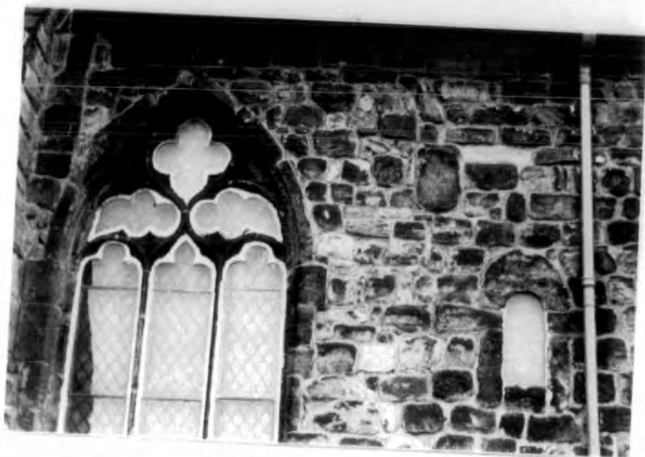
South wall exterior: upper doorway
