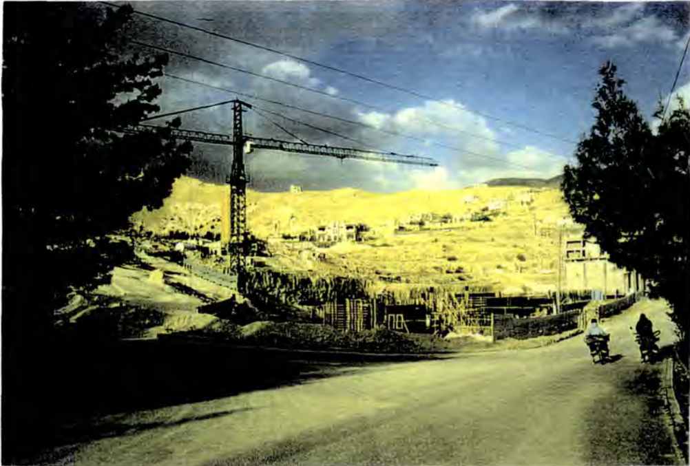
Figure 7.10 Hotel construction site in Petra in 1994
