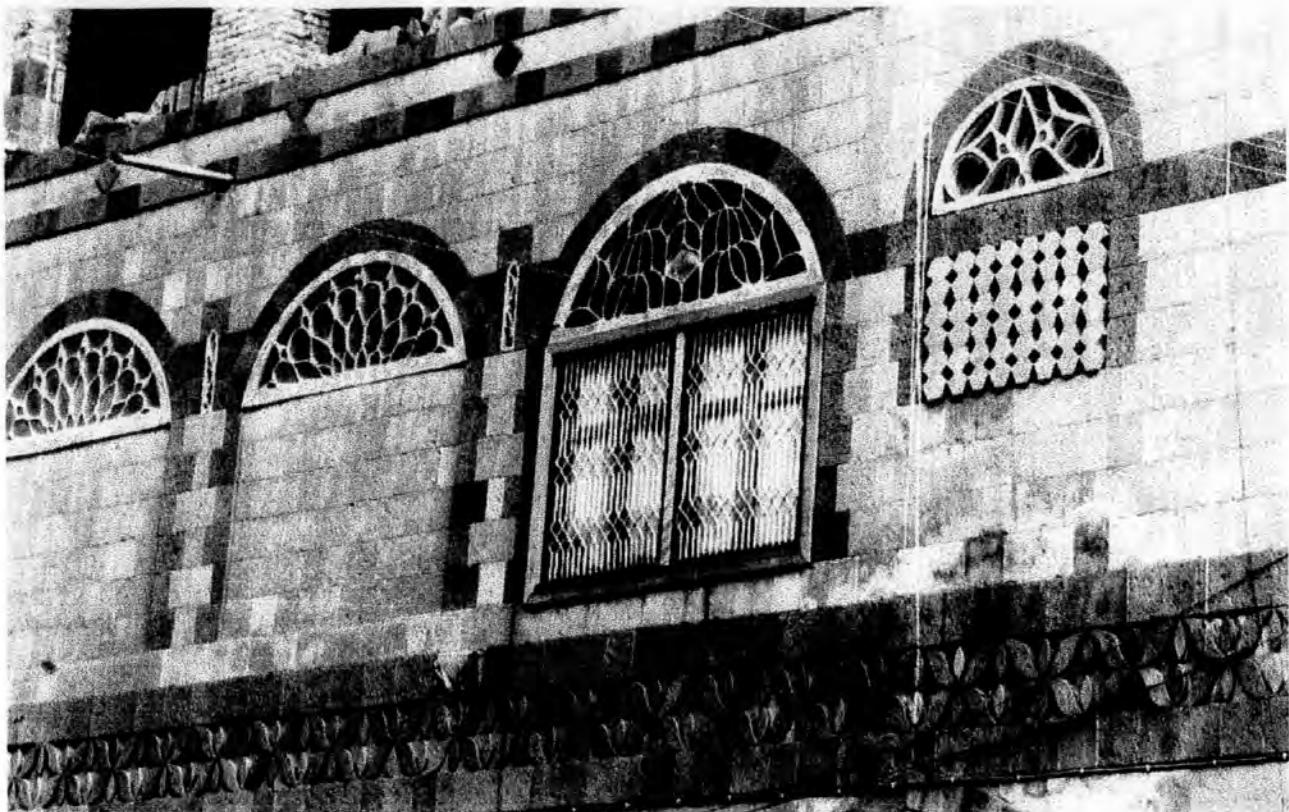
Stone work in the early 'seventies by a mason of traditional Sana'ani extraction ( top ) and by a migrant mason ( bottom )
