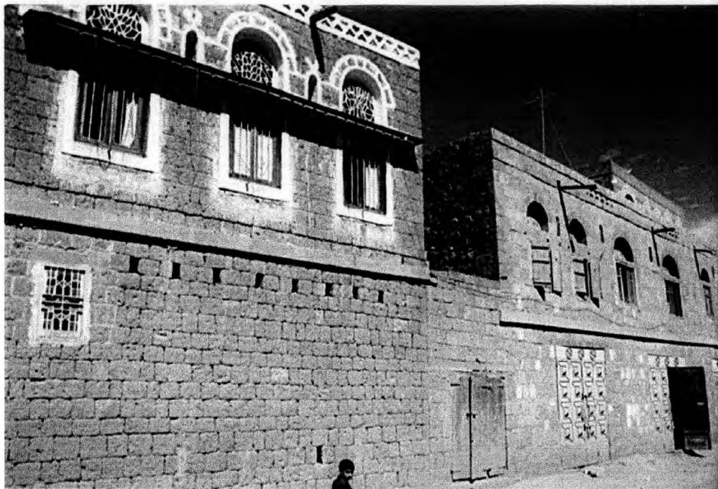
Top - Reinforced concrete lintels introduced in stone houses after the earthquakes, Dhamar; bottom - Construction in Dhamar, 1990
