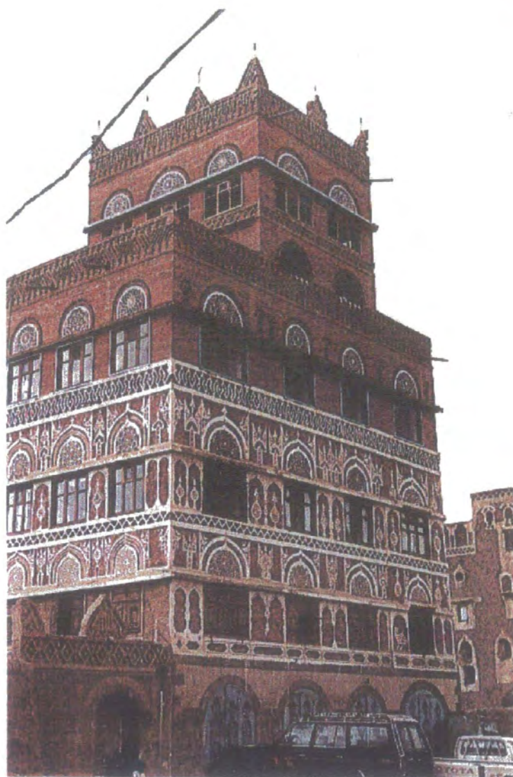
Top - Recent construction in handcrafted baked bricks, Al Rhawdha; bottom - Industrial bricks, Sana'a, 1990
