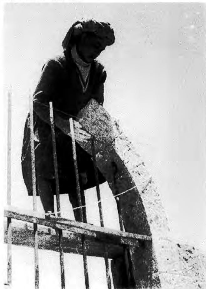
Top left - Children's construction, Wadi Dahr; right - Plasterer and helper; bottom left - Cantilevers and wood brackets in Thula; right - burglar bars as formwork
