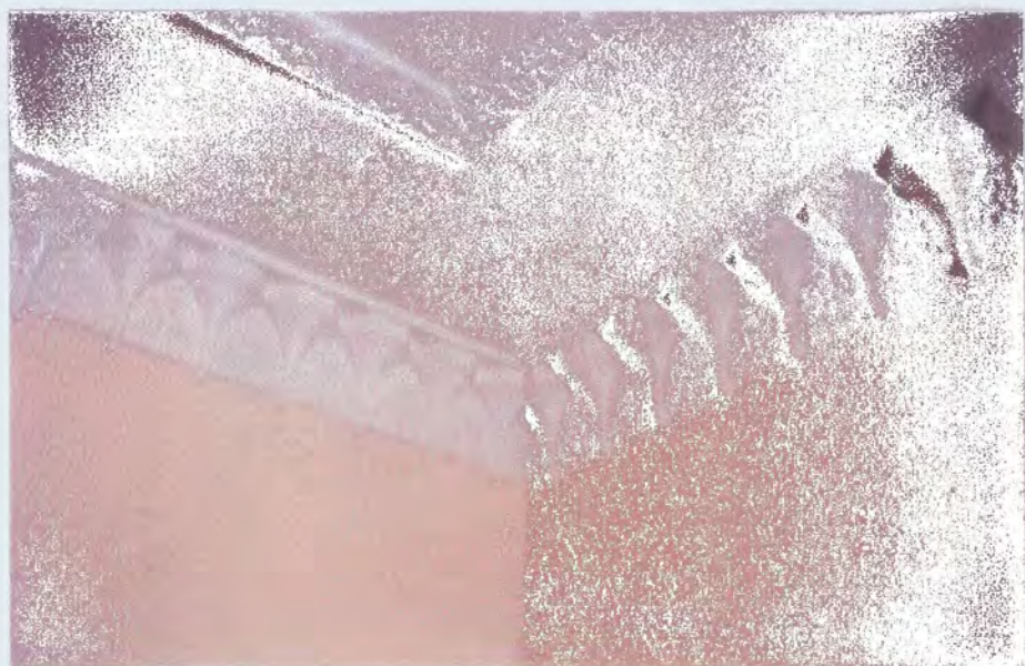
Top left- New maqraj rendered with cement and painted enamel, Mithal; right, centre and opposite - Carvings in new gypsum plaster rendered maqraj, Sana'a; bottom - Mouldings, Sana'a
