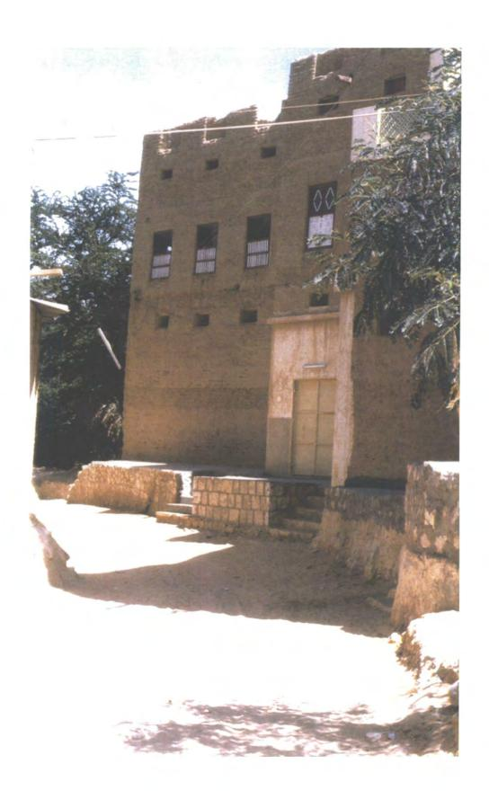
Plate 2. Substantial foundations used for a house on the edge of a channel in Tarim.
