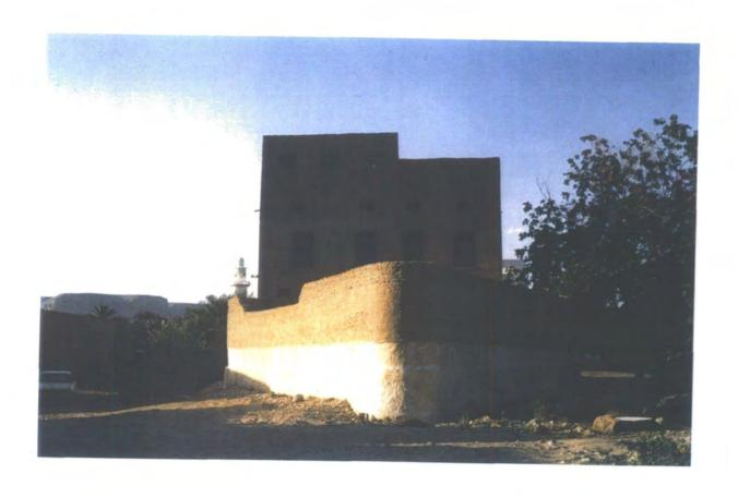
Plate 6. Building No. 1, Built between two water- courses, this house needs massive foundations
