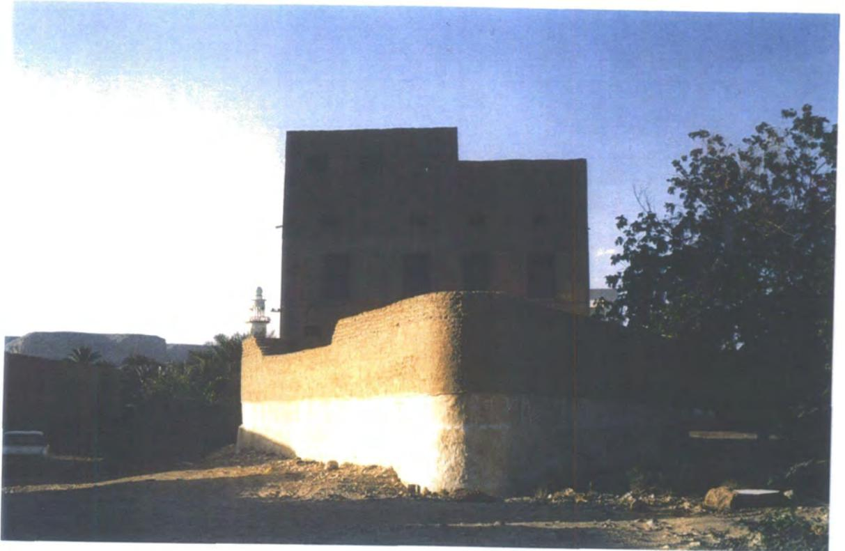
Plate 6. Building No. 1, Built between two water- courses, this house needs massive foundations
