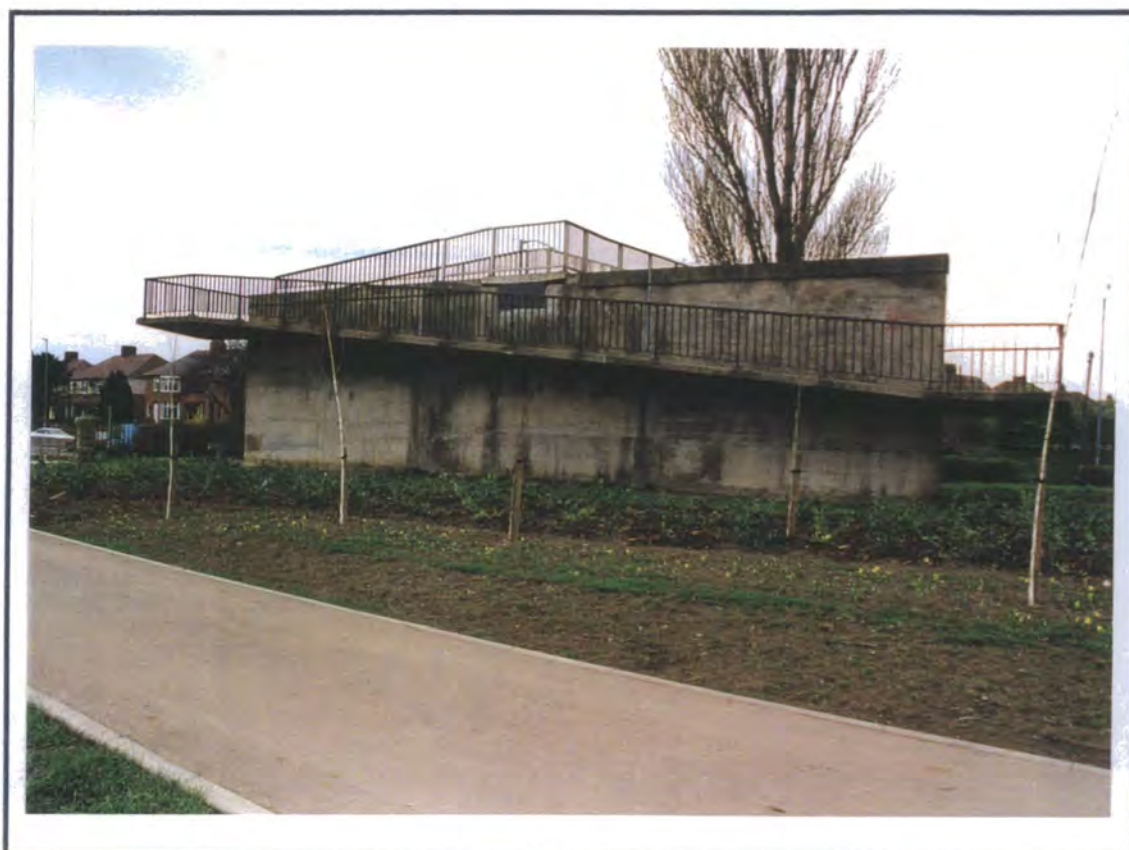
Fig. 5.11 Footbridge Crossing A167(T) Showing Restricted Visibility.
