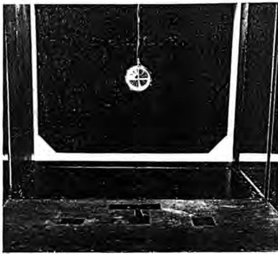
Figure 7 Photograph showing field mill in the lower foreground with the ion generator above.
