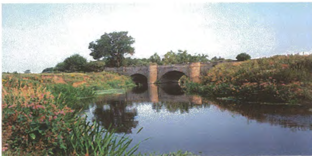
Figure 2.15 Nidd at Skip Bridge. Looking downstream towards the bridge. Light attenuation readings were taken from the near bank.
