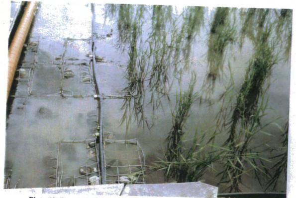
Plate 13. Flooded rock-gabions and pot-grown *Phragmites australis* inlet section of the CATS Terminal reedbed, 14.00 hours, 1/7/97.
