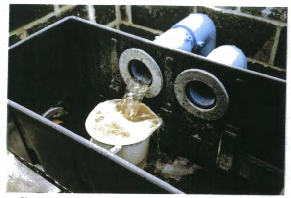
Plate 3. Wastewater inlet tank at the CATS Terminal reedbed, January 1997, showing secondary treated effluent entering the system from the Klargester.
