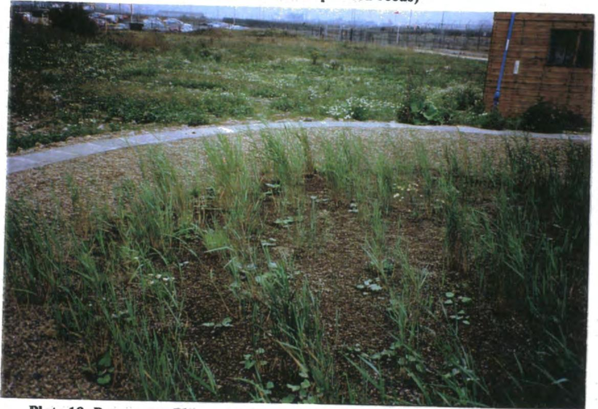
**Plate 18. Pot-grown *Phragmites australis* outlet section of the CATS Terminal reedbed, August 1997, showing shoot-density and height of reeds.**
