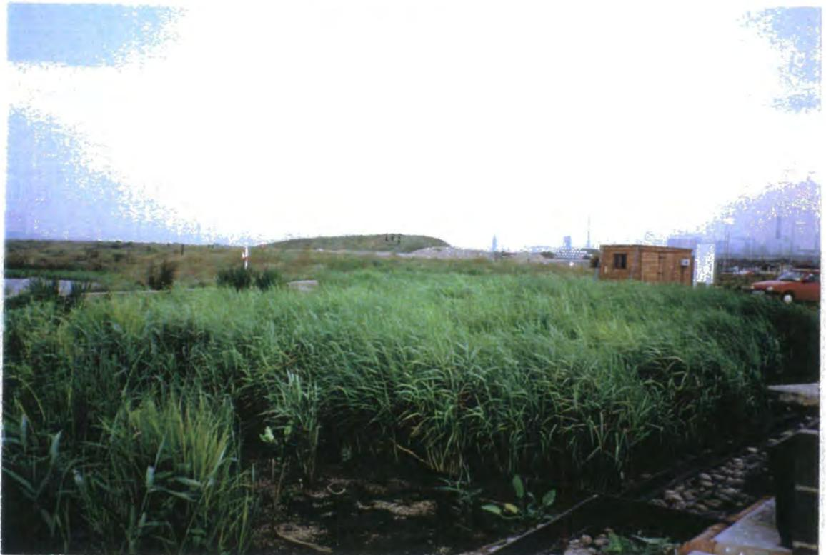
**Plate 12. Pot-grown *Phragmites australis* section of the CATS Terminal reedbed, late August 1997. (Local reed inlet section in the foreground showing less successful establishment of planted reeds)**
