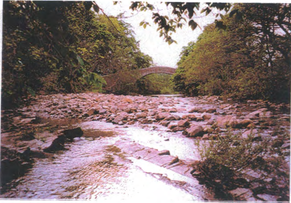
Figure 3.9 R. Swale at Ivelet Bridge, km 10.9 (June 1996)
