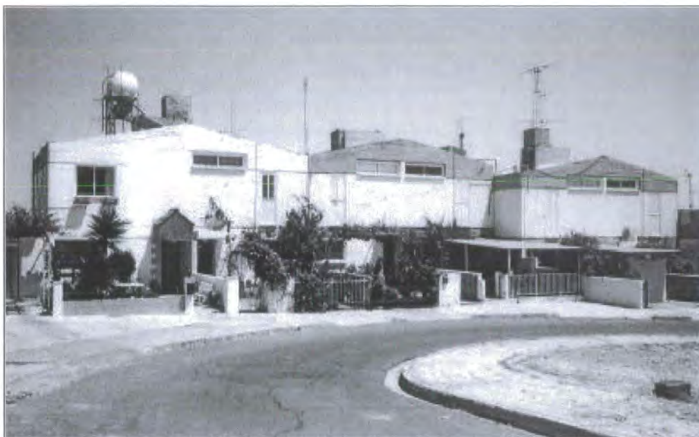
The house on the left of this picture, has recently undergone investment after the owner received title for his property. New windows, an extension (on the far left) and a new roof-mounted heating system have all been added. Other houses retain the appearance they had when they were first constructed.
