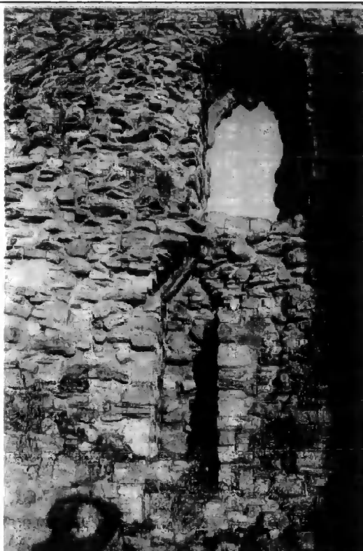
Plate 9 A Triangular Headed Mural Passage in the East Curtain Wall of Richmond Castle
