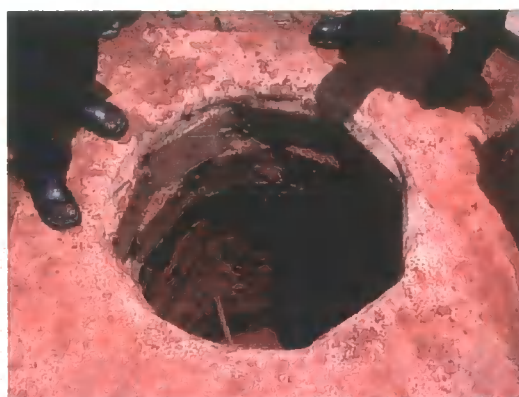
Figure 6.5 Completed latrine 'collar' ready for digging
