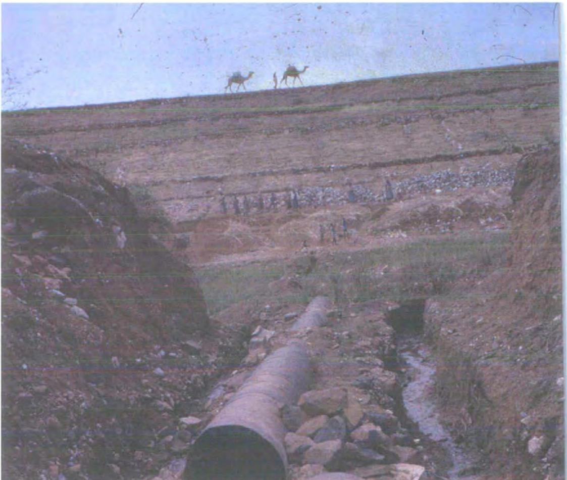
Plate 4.1. The seepage area and the dam embankment seen from below.
