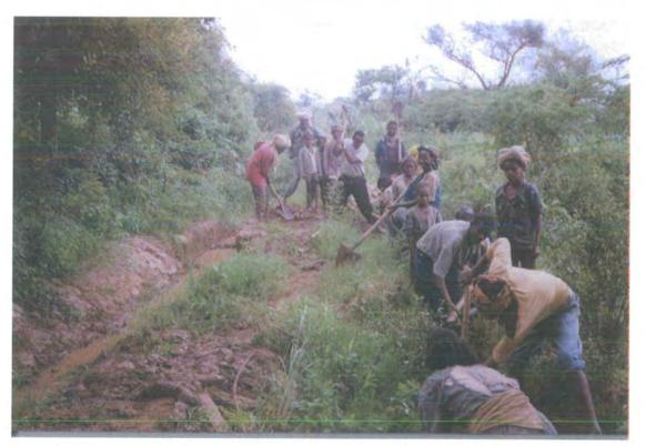
Plate 6.1. Digging a drainage canal (below) and a crossing canal (above) to cultivate more land on the other side of the gully below the dam.
