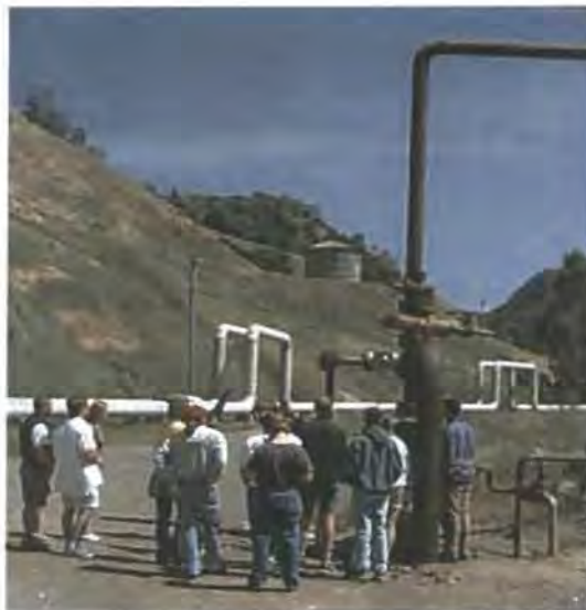
Figure 1.28: An injection well at The Geysers geothermal area. Most injection wells are located in the vicinity of the power plants. (from : http://corporate.stanford.edu/research/programs/geoth.html )
