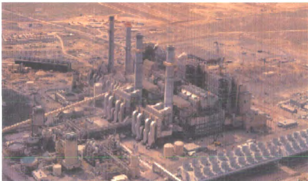
Illustration 1 World's largest regenerable FGD unit
